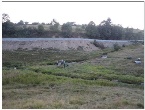
Figure 5: Loose slopes, on the roadside of Brebu-Slatina Timiş near the Lung Stream, increase sedimentation and habitats degradation impact on salmonids.
