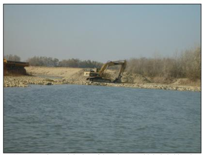
Figure 23: Aggressive exploitation of the substrate with lotic habitat damage.
